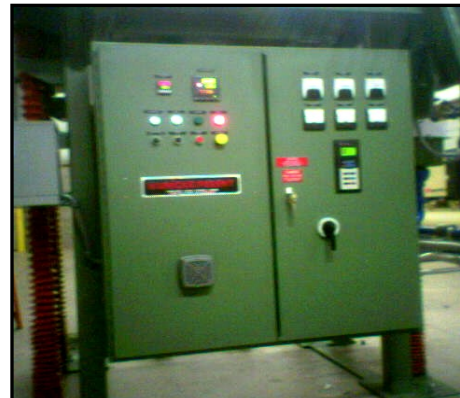
Operator Friendly Control Centers
